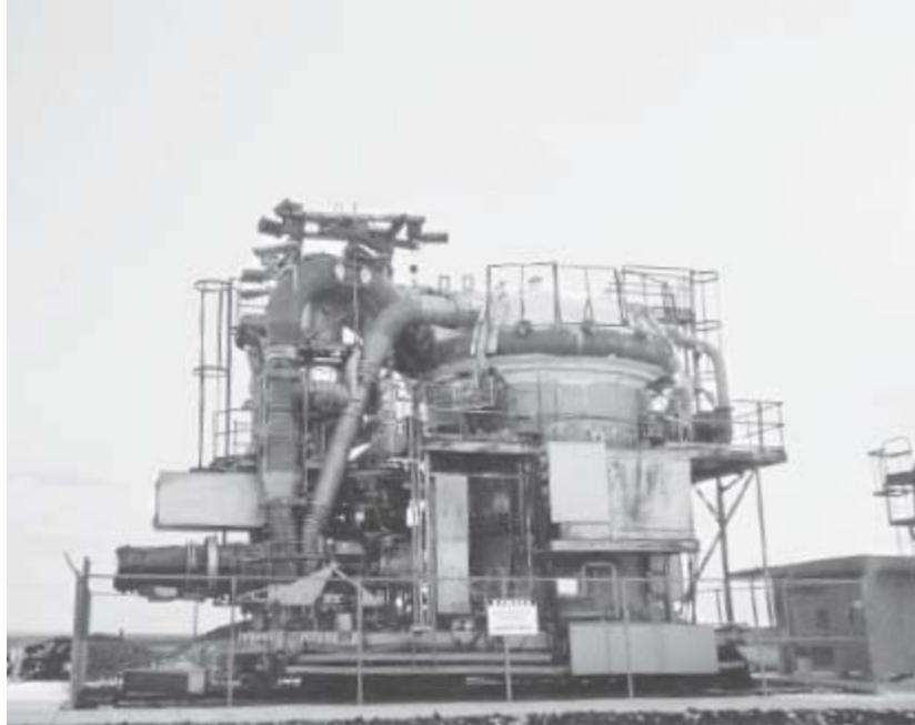
The Air Force HTRE experiments joined a nuclear reactor to two General Electric J-47 jet engines. (Todd Tucker)
